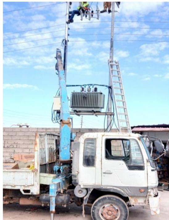
Transformers are installed and connected to the poles.
